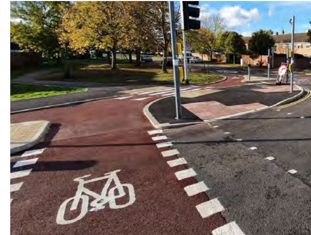
Figure 2: Example of a major junction improvement, Cambridge
