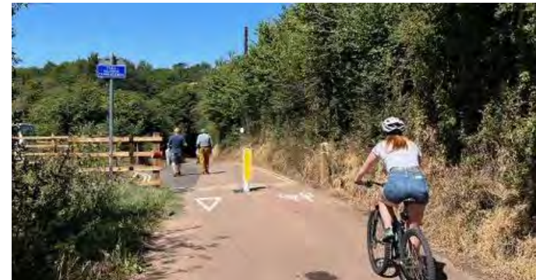
Figure 2: Example of a shared use path, Ludwell Valley Park, Exeter
