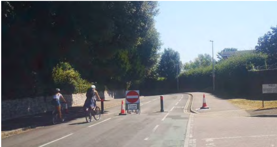
Figure 7-1 - Temporary modal filter on the E9 cycle route, Dryden Road
